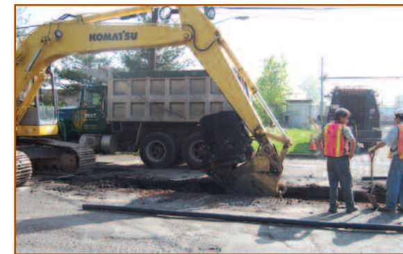
The Vera Cruz sewer project is moving forward.
