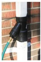
3. Direct the overflow tube away from your foundation. You may set the end of the tube inside a piece of corrugated gutter, under rocks, to a vegetable garden or it could even lead to a rain garden!
