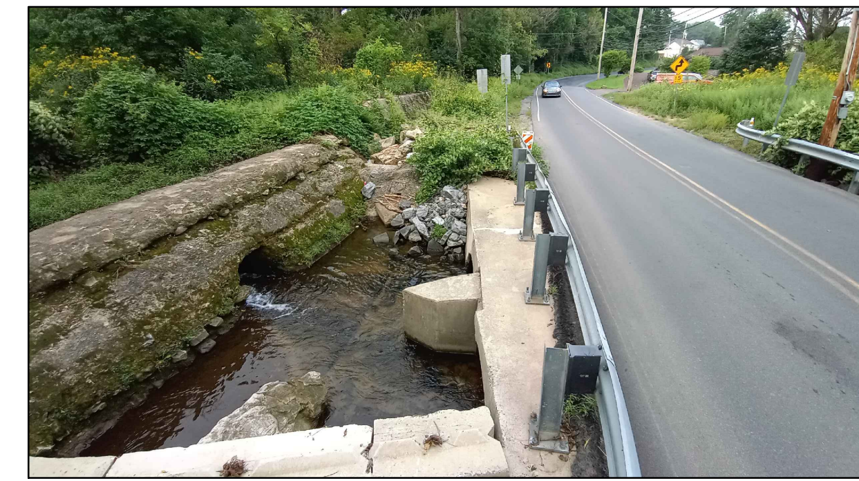
SR 2018 (LOOKING WEST)
